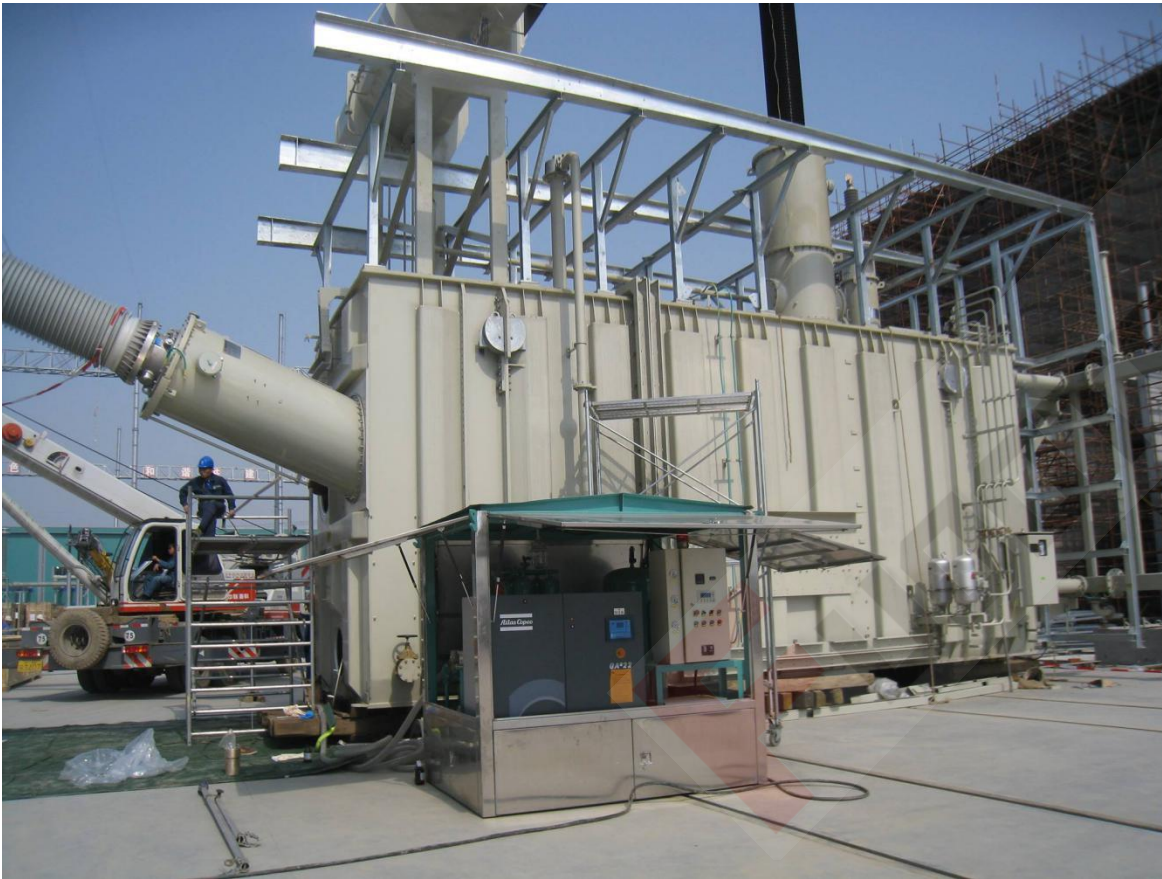
FUOOTECH Transformer Drying Air Generator for transformer maintenance
